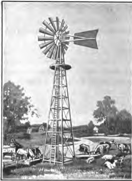
FIG. 182. — The windmill pumps water into the troughs where cattle drink.
